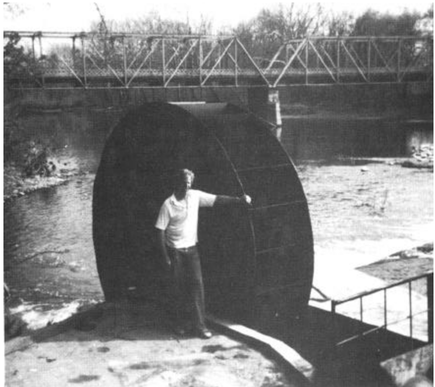
A FITZ Waterwheel Company all-welded steel undershot wheel.
